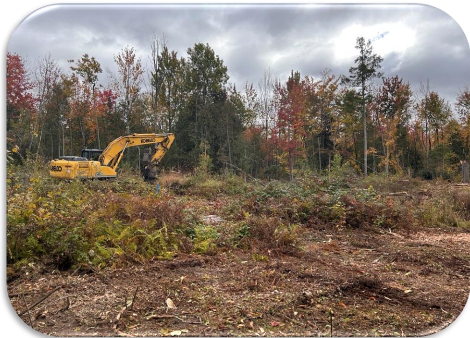
Site prep for fall 2024 planting Private site in Alfred-Plantagenet
