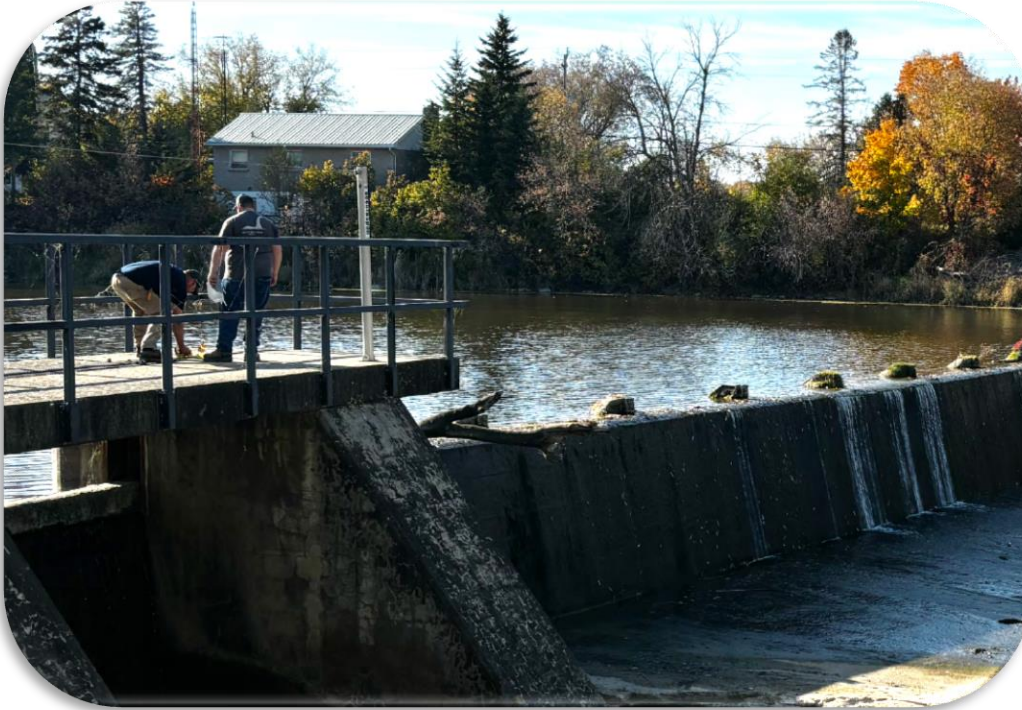
Crysler Dam Inspection – October 2024
