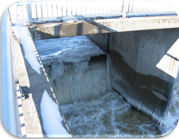
Ice forming in stop log bay – Chesterville Dam, Jan 2014
