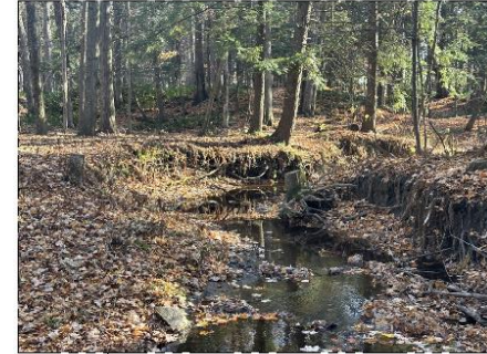
Downstream of Coir Logs & Log Vane.
