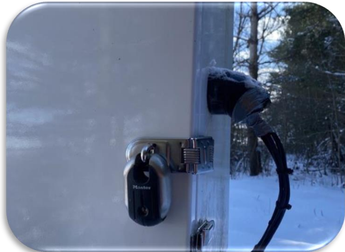
Pleasant Valley station – new lock installed
