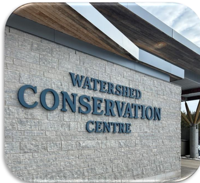
Tour of Upper Thames River Conservation Authority LEED Platinum Office Building
