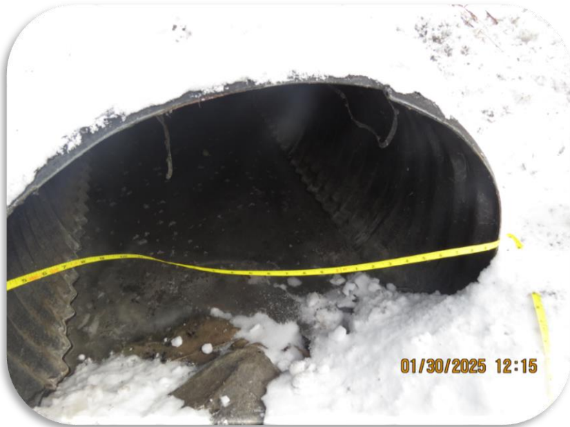
Permit inspection for a culvert replacement City of Ottawa
