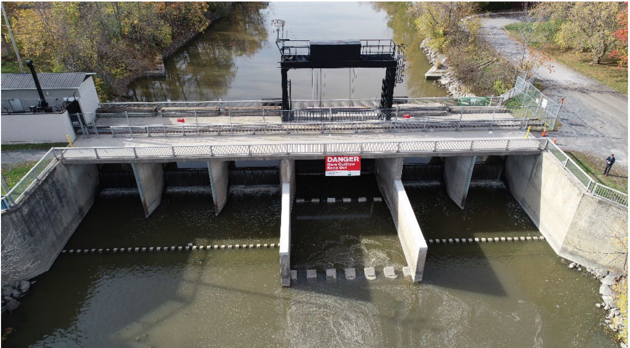
Figure 17. Chesterville Dam photo in Chesterville, Ontario.
