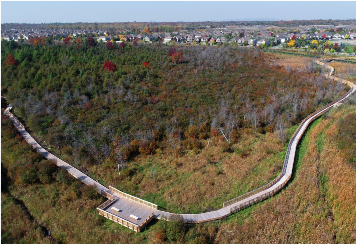
Figure 1412. Findlay Creek Boardwalk, City of Ottawa, Ontario.
