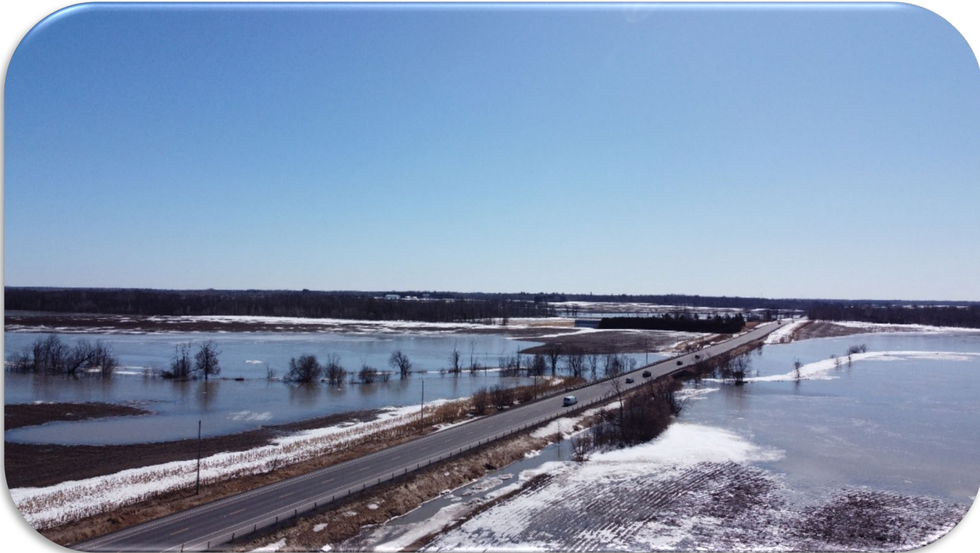
Bear Brook flooding at Frank Kenny Road in the City of Ottawa
