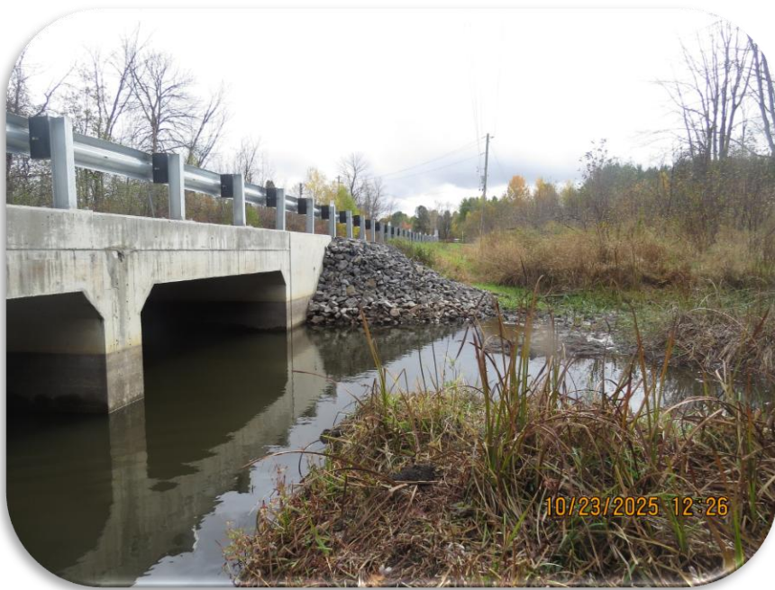
Culvert replacement and erosion control works on County Road 44, Edwardsburgh Cardinal
