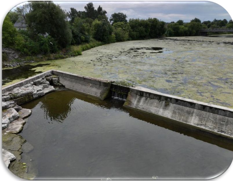
Drone image of Casselman Dam sluiceway August 2025
