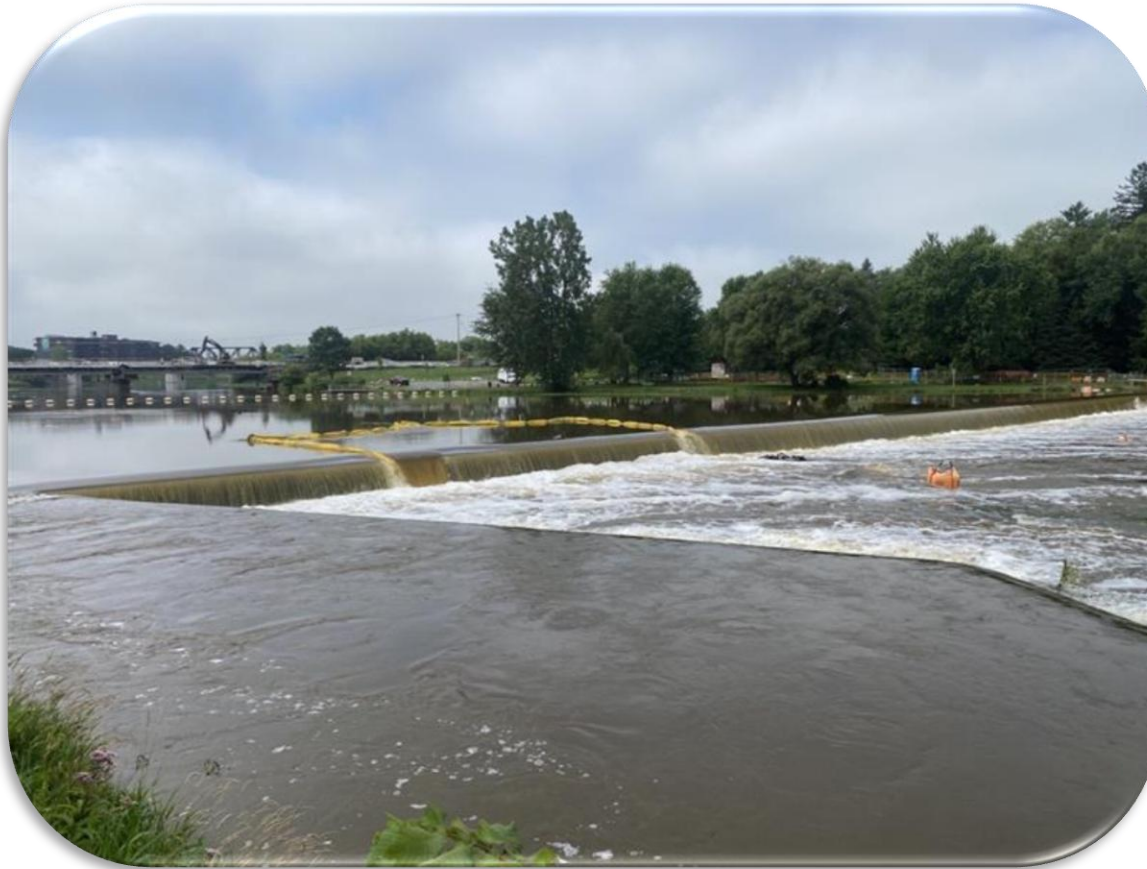
Casselman Dam – July 31 st
