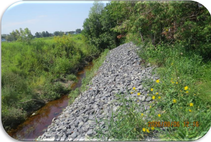
Erosion Protection in the Nation Municipality
